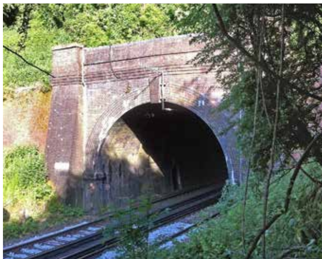
South portal of Oxted tunnel
